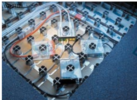
The specifically for use with Intercell cable management floors developed COMBIbox model.
