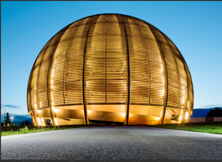
HIGGS BOSON FACILITY CERN SWITZERLAND
